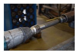
5 Remove long screw socket, if possible apply plastic mortar around the end of the Thorbolt / entrance of the drill hole, fit the dome plate, hemisphere and nut. Buckle up ditto. (**Note**: If plastering cannot take place in this step, it must be carried out in connection with step 7, grouting)
